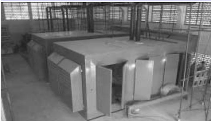
The **Power Generation Plant** as seen above was commissioned on March 31, 2003. The power plant houses two 1.5 megawatt natural gas powered generators along with two standby diesel generators, 1.0 megawatt each. The plant is now operational supplying economical power to over 60% of the campus. ■
